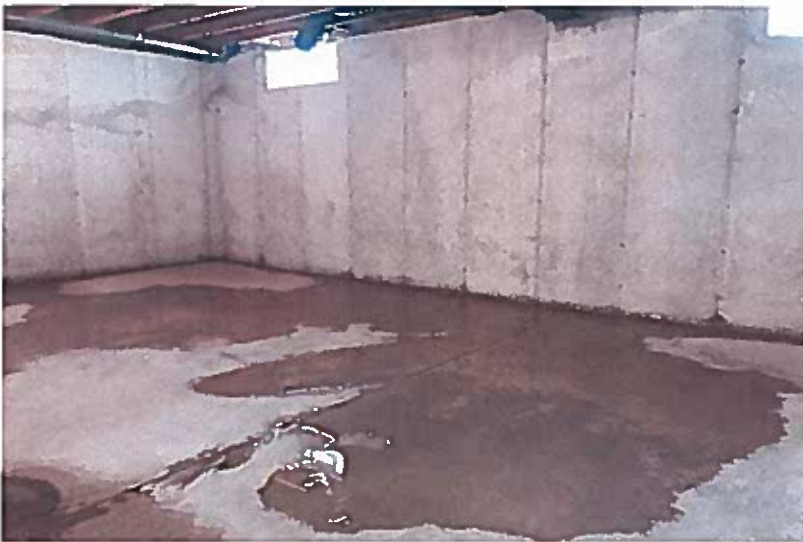
Water seepage after only a couple hours of rain
