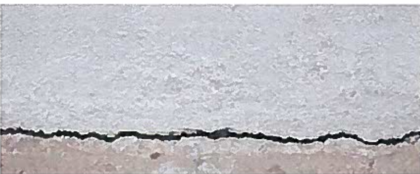
Crack in foundation – roughly 14 inches long
