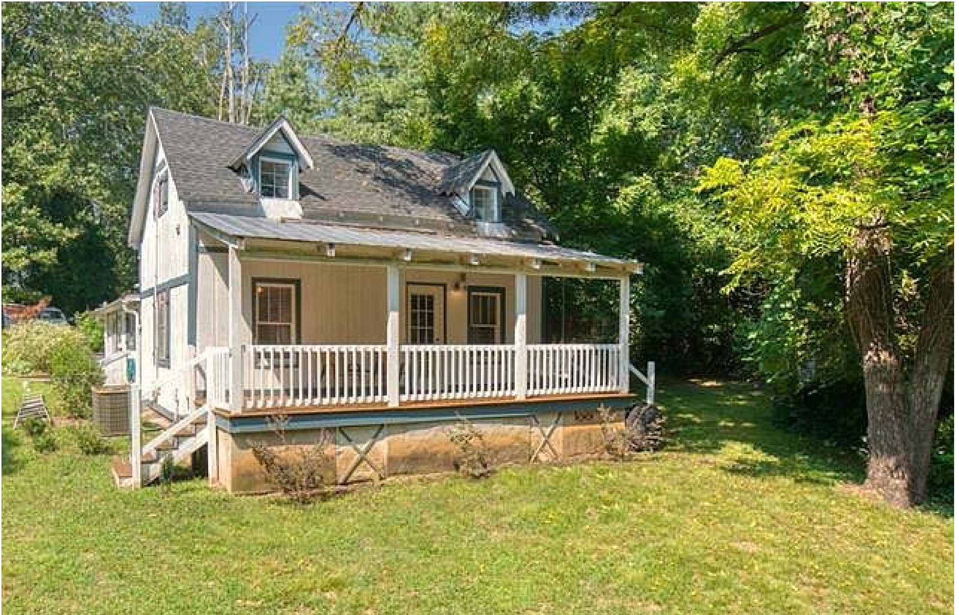
Front of subject house 6819 Elm Street June 17, 2019
